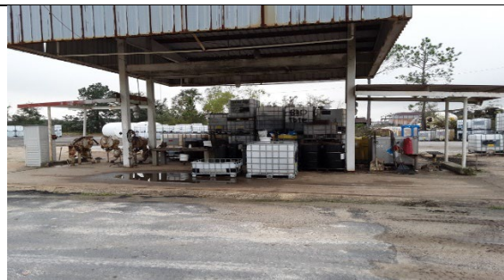
Photo-24 Housekeeping and Container Management addressed at the Canopy
