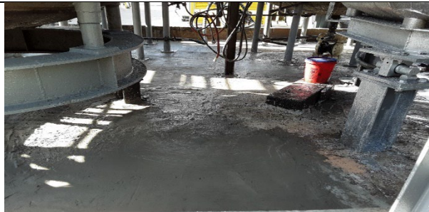
Photo-11 Production Area #3 Partial Resurfacing of the containment Floor
