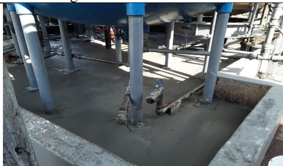
Photo-12 Production Area #3 Partial Resurfacing of the containment Floor
