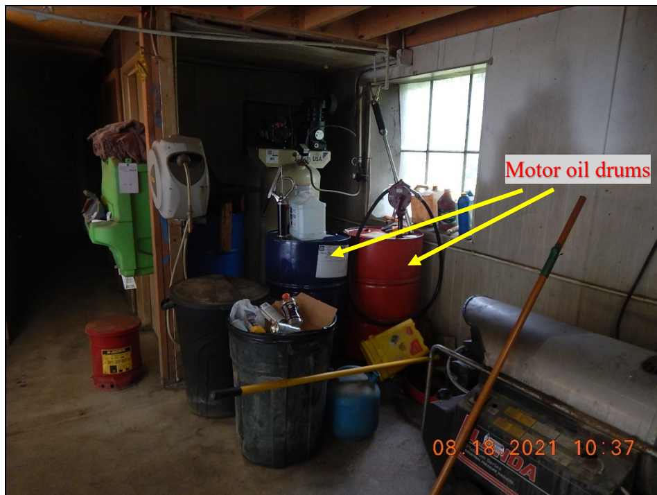
Photograph 30. Municipal Garage: (DSCN0730) View of two 55-gallon drums containing motor oil and other small chemical storage. Note that the 55-gallon drums were not located on spill pallets or within secondary containment; however, an oil spill kit was located inside the municipal garage.
