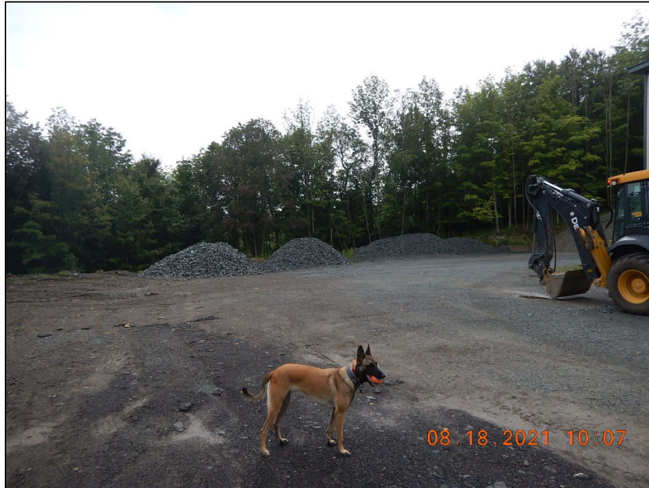
Photograph 25. Municipal Salt Storage Shed: (DSCN0721) Alternate view, facing east, of crushed stone piles behind the salt storage shed.
