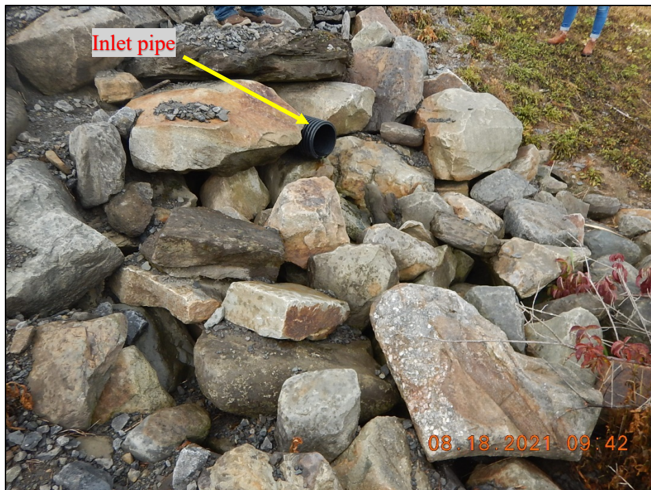
Photograph 18. Francis Smith & Sons Detention Pond: (DSCN0710) View, facing west, of the inlet pipe from the parking lot to the east detention basin. Note the rip rap surrounding the pipe opening.
