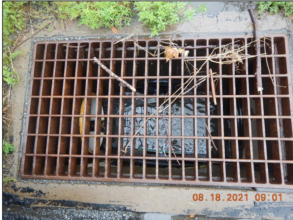
Photograph 3. Outfall #2: (DSCN0700) View of the closest upgradient inlet from Outfall #2.
