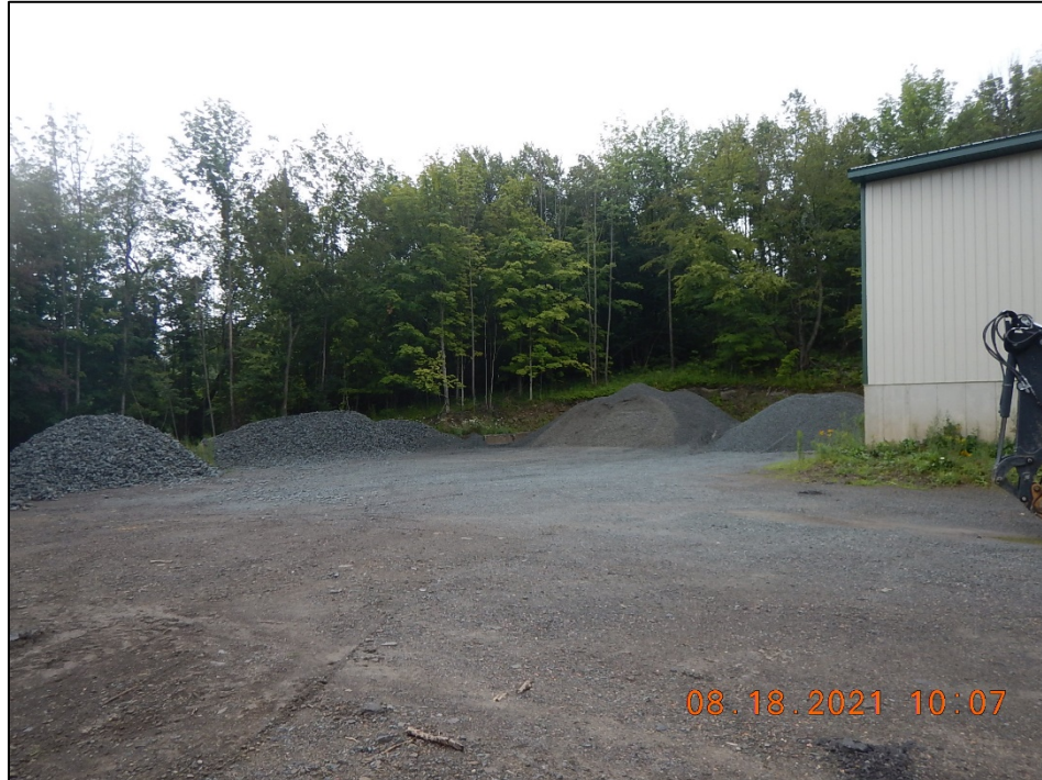
Photograph 24. Municipal Salt Storage Shed: (DSCN0722) View, facing southeast, of four crushed stone piles behind the salt storage shed. Note the lack of cover and impermeable containment.
