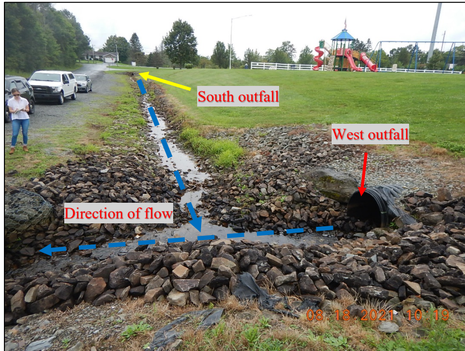
Photograph 11. Municipal Park Outfalls: (DSCN0723) View, facing south, of the south outfall discharging to a ditch and merging with the outfall ditch from the west outfall.
