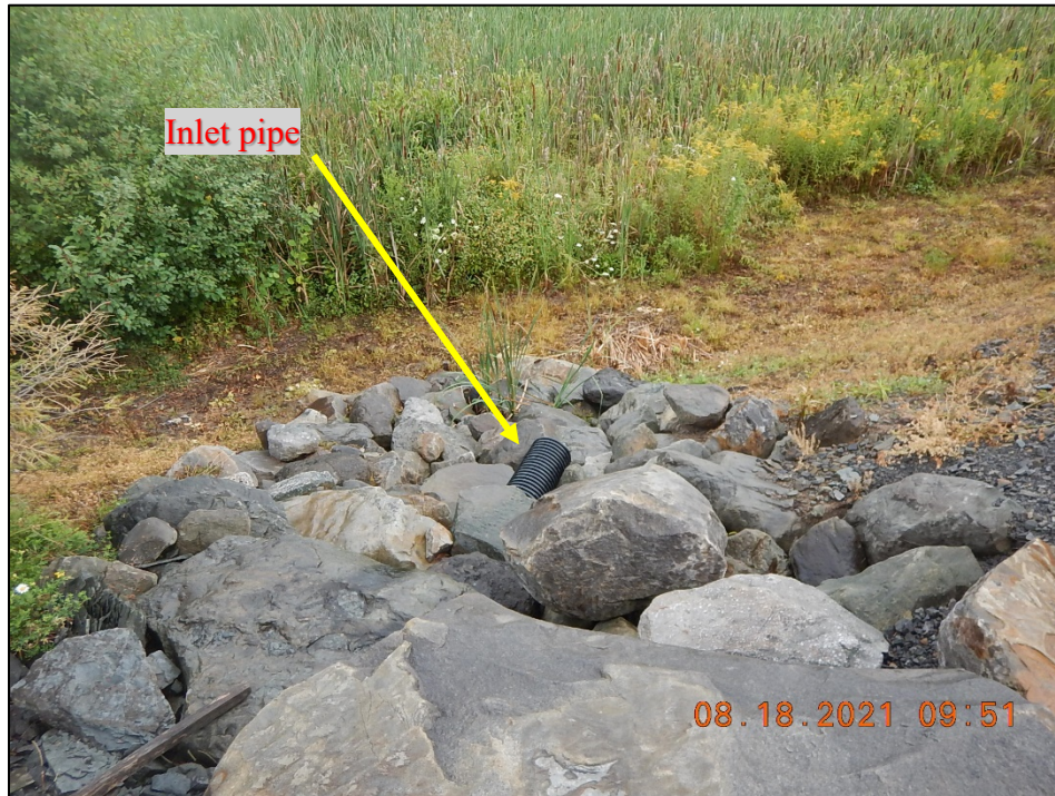
Photograph 21. Francis Smith & Sons Detention Pond: (DSCN0717) View, facing north, of the inlet pipe from the parking lot to the west detention basin. Note the rip rap surrounding the pipe opening.
