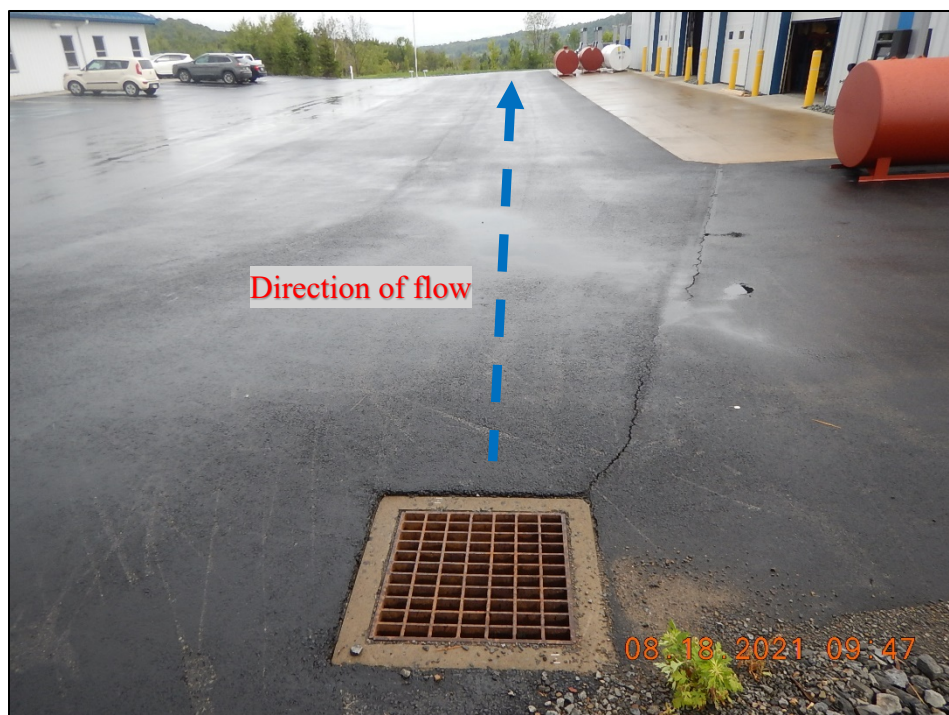
Photograph 20. Francis Smith & Sons Detention Pond: (DSCN0716) View, facing north, of the parking lot uphill of the west detention basin. Note the presence of an inlet flowing to the west detention basin.
