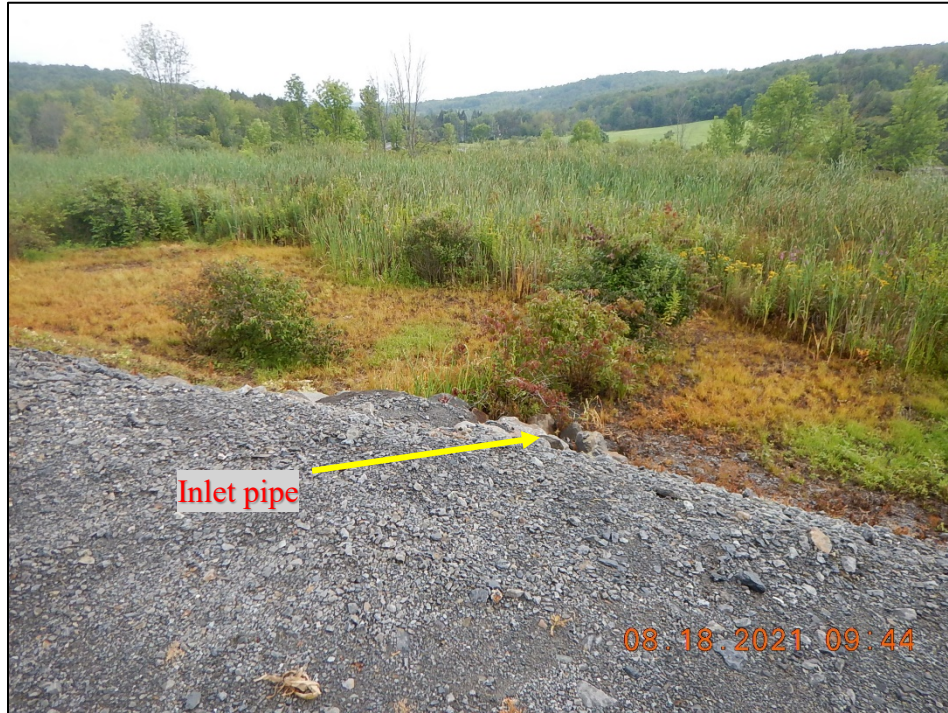
Photograph 17. Francis Smith & Sons Detention Pond: (DSCN0713) View, facing north, of the east detention basin, located approximately 20 feet downhill from the parking lot.
