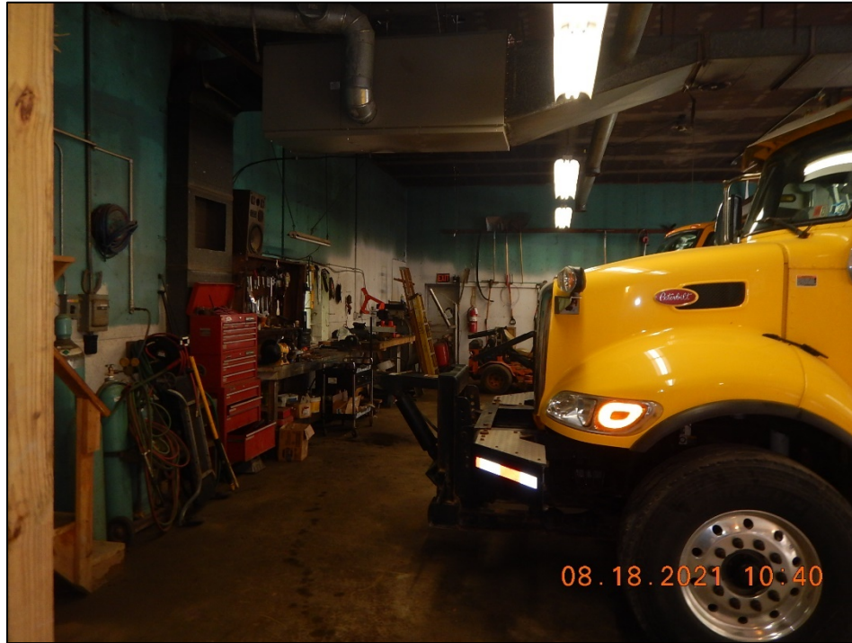
Photograph 29. Municipal Garage: (DSCN0731) View of tool storage inside the municipal garage.
