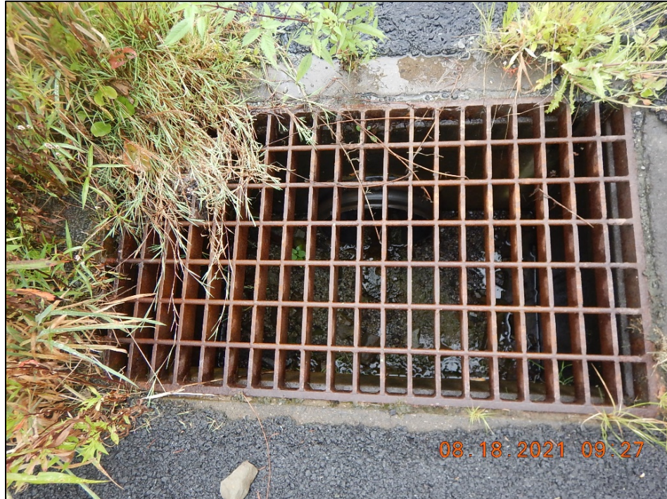
Photograph 10. Hill Street Outfall: (DSCN0709) View of the only upgradient inlet piped to the Hill Street Outfall, located approximately 20 feet west of the outfall. Stormwater runoff was observed going into the inlet at the time of the inspection.
