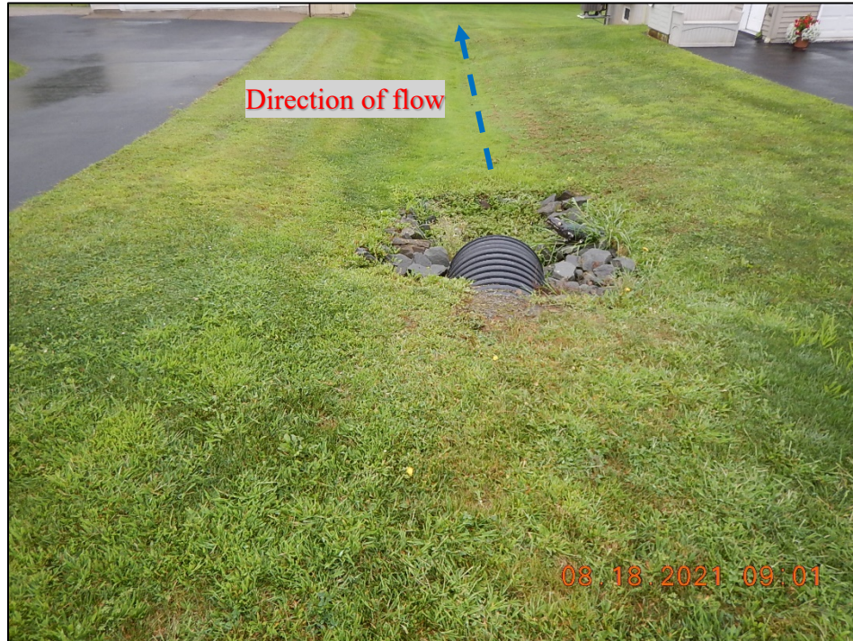
Photograph 1. Outfall #2: (DSCN0701) View, facing south, of the end-of-pipe labelled Outfall #2. The outfall discharges to a grassy ditch between two houses, which connects to a tributary to Leggetts Creek, approximately 300 feet to the southeast.
