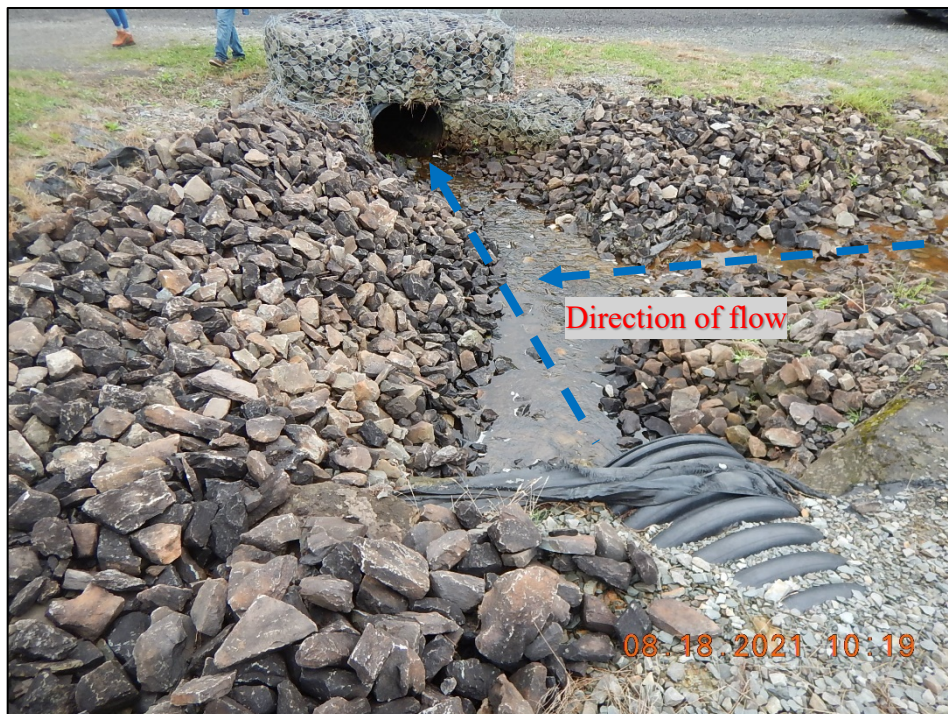
Photograph 12. Municipal Park Outfalls: (DSCN0724) View, facing east, of the south and west outfall ditches merging and flowing under Mostowski Road.
