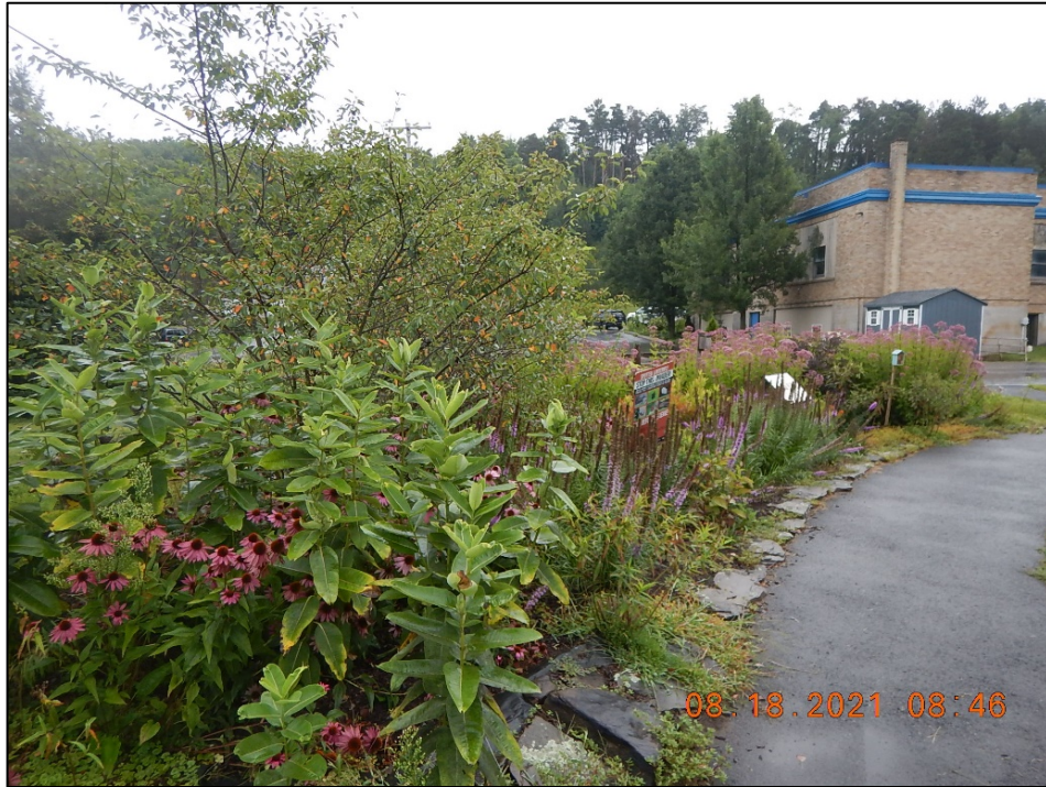
Photograph 15. Municipal Building Rain Garden: (DSCN0696) View, facing northeast, of the municipal building rain garden. Note the Scott Township Municipal Building and parking lot in the background.
