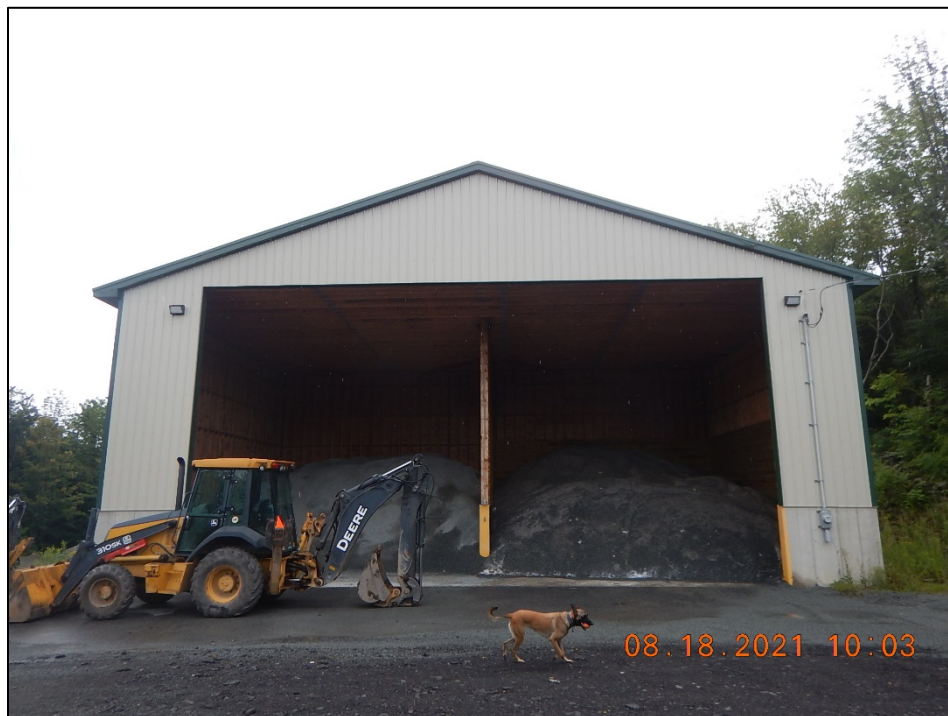
Photograph 22. Municipal Salt Storage Shed: (DSCN0719) View, facing east, of the municipal salt storage shed.
