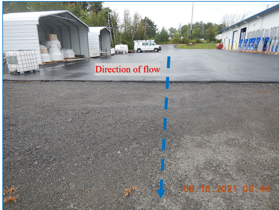
Photograph 19. Francis Smith & Sons Detention Pond: (DSCN0714) View, facing south, of the parking lot uphill of the east detention basin.
