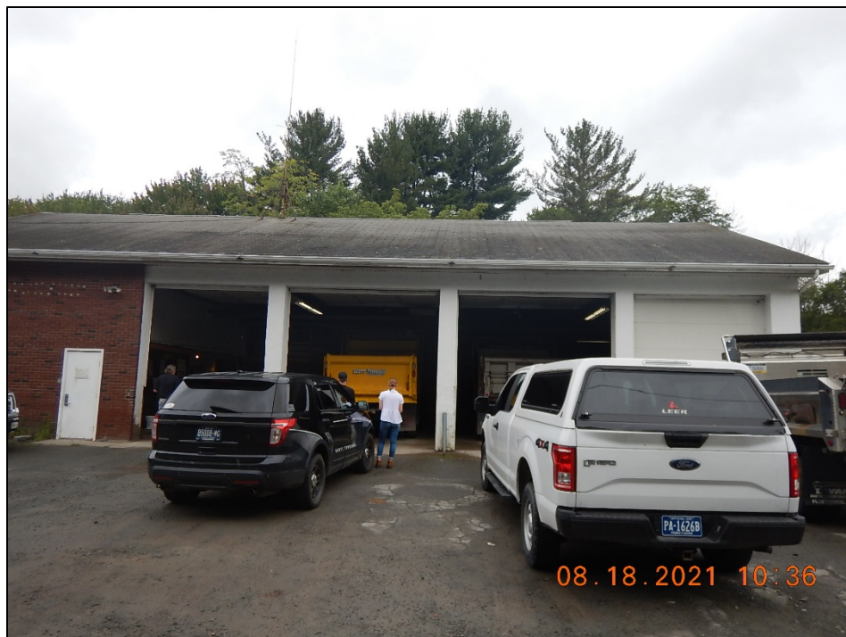
Photograph 26. Municipal Garage: (DSCN0728) View, facing west, of the Municipal Garage and gravel parking lot.
