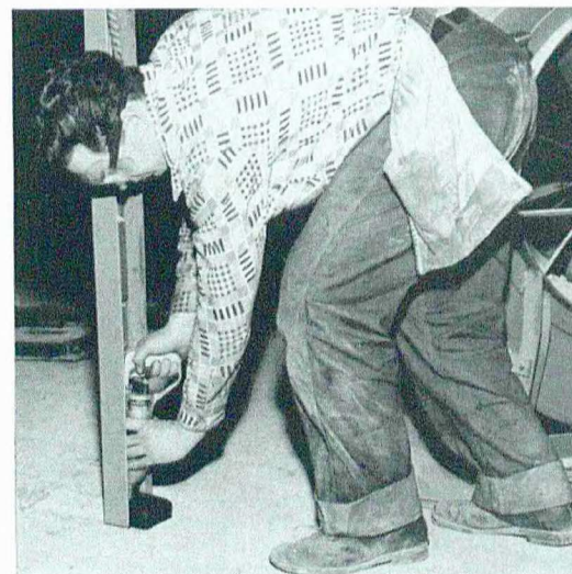
Here Remington Stud Driver fastens a steel door buck to concrete. Speed is tool's big advantage.
