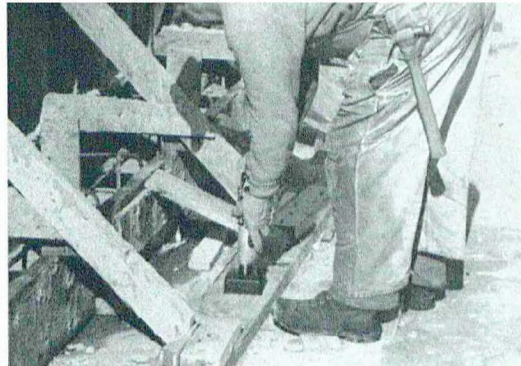
Form shoring is anchored to concrete with Remington Stud Driver. Tool is completely portable.
