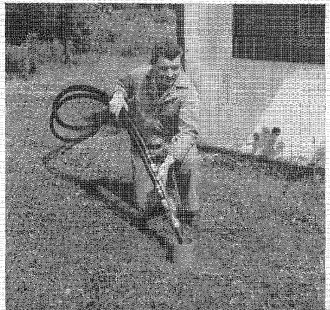
Simplicity of installation is major virtue of lightweight pipe of "Alathon". Since it's flexible, it can easily be snaked around obstacles and laid at uniform depth regardless of land contours.
