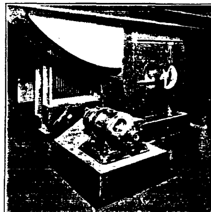
Fan and Motor Installation
