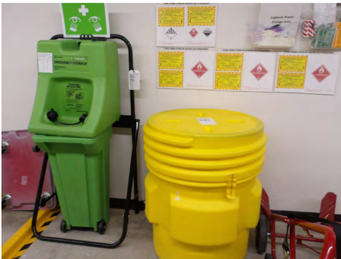
Photograph Two (2): Eye washing station and spill kit
