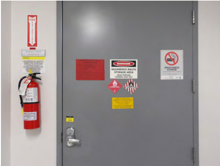
Photograph Three (3): Outside view of the CAA
