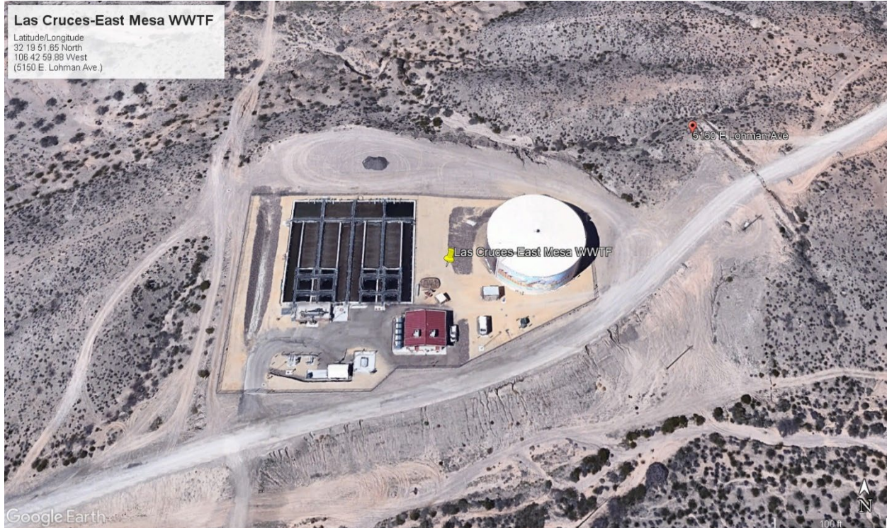
Aerial Image #1: Overall view of the City of Las Cruces' - East Mesa Wastewater Treatment Facility. Aerial from Google Earth maps.
