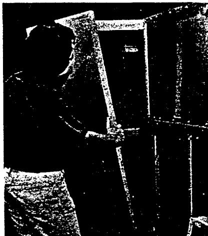
Panels can easily be installed by one man without the use of mechanical materials handling equipment
