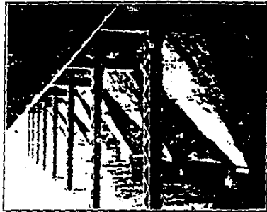
Basic Sulphate White Lead—Hoppers Under Collecting Bags
