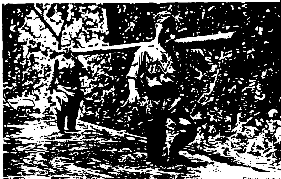
To build the CBI pipeline, the crews often worked waist-deep in water, stringing and coupling the pipe
