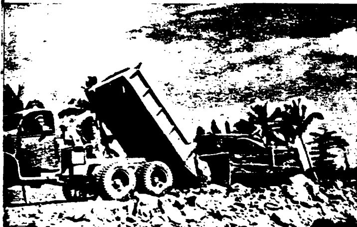
In record time, the Seabees built a four-lane superhighway on Guam, equal to any in the U. S.
