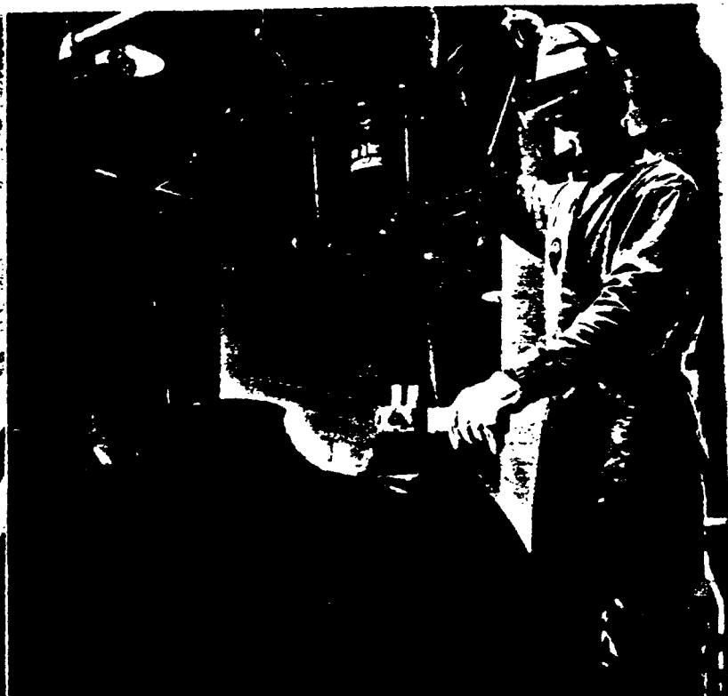
The woman at the left is inserting a booster charge into a bomb, after a workman, right, pours in molten TNT, the main explosive
