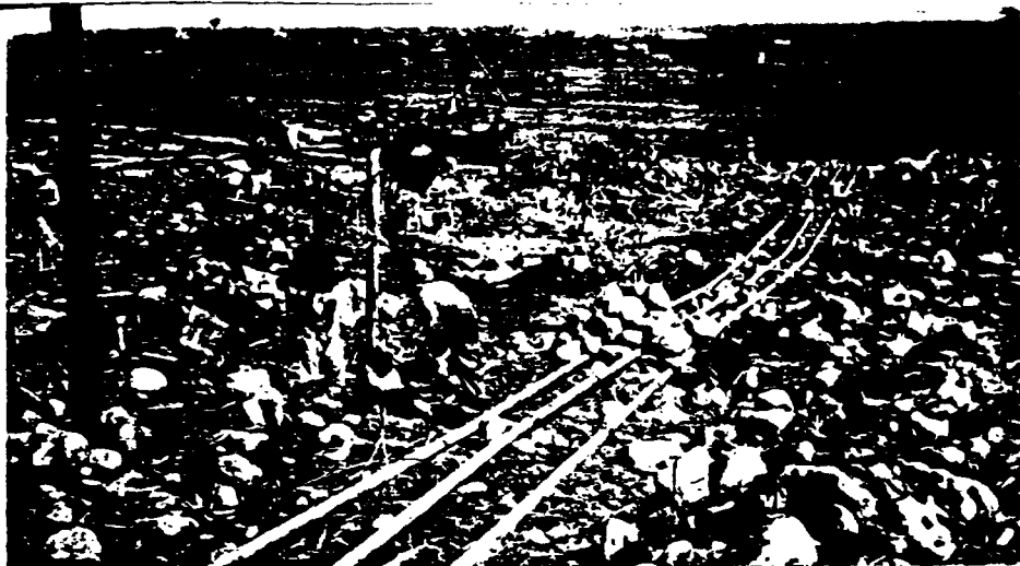
These pipelines were hastily laid to power the push across Iwo Jima. They are typical invasion pipelines
