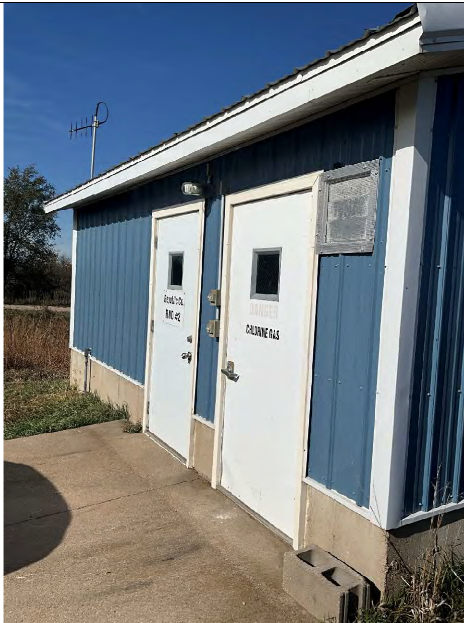
View of the exterior of the South Well house
