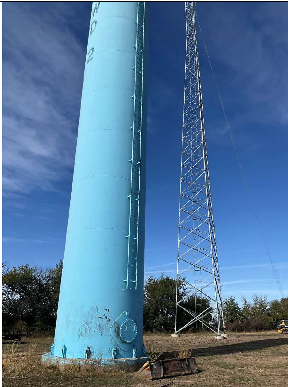
View of the Francis Tower adjacent to communication tower
