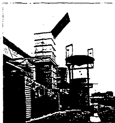
Fig. 13. (L to R) Filter houses for test stands on roof of building. Exhaust stack stand, filter house and exhaust stack stand in process of erection
