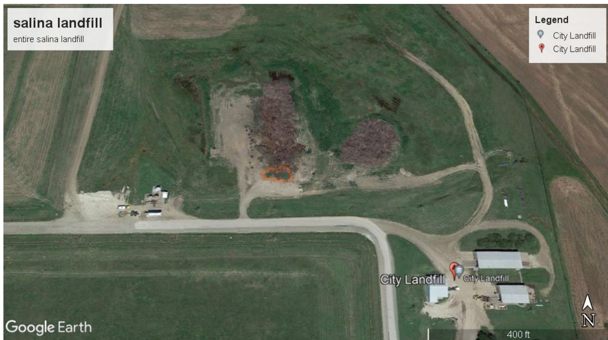
Figure 1. On-site burning area
