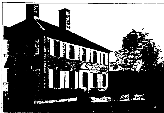
The Marion Litchfield residence at Bedford Village, N. Y. has lead ridges, hips and chimney flashing. Godwin, Thompson and Patterson, New York, architects.
