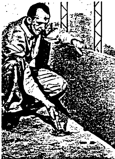
FIRST COURSE of BAXBORD base is placed against studs and locked in place with TRUS-LOK TL-2 starter clips, which also secure the top course.
