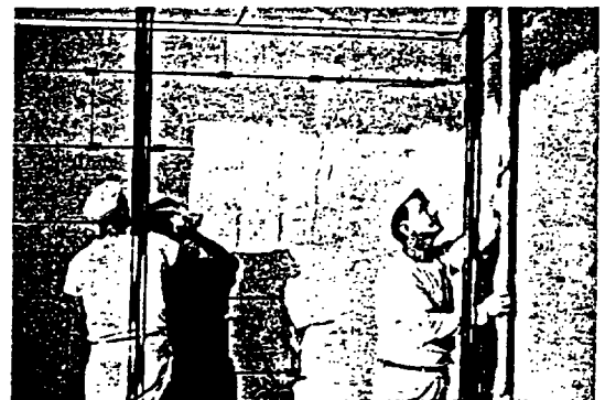
THE TRUSSTEEL STUD SYSTEM works equally well with a plaster facing. The ROCKLATH plaster base is clipped to the studs in the same manner as the BAXBORD base.
