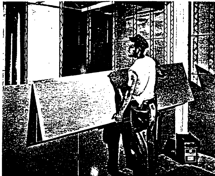
EASY-TO-HANDLE BAXBORD panels are set in the upper flanges of the butterfly-shaped TL-1 clip which holds the preceding course in place. Notice that joints are allowed to fall between the studs.
