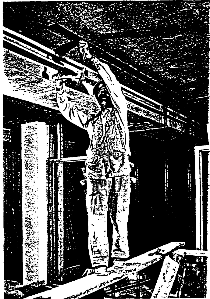
STANDARD STEEL-RUNNER TRACKS are nailed in place along partition lines marked on both the floor and ceiling slabs.
