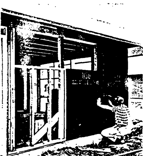
BIG SHEETS of USG Insulating Sheathing make fast work of closing in a house. It has good racking strength and insulating properties.
