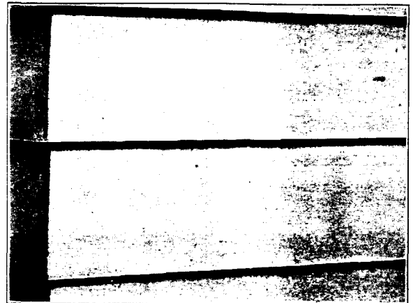
Detail of the paint on the exterior of the Gordon home, showing the perfect condition of the white lead after three years' exposure.
