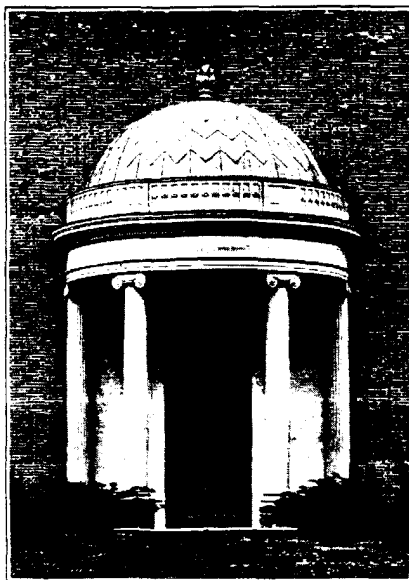
Lead-roofed entrance to a private tennis court. Note design of seams. DELANO & ALDRICH, ARCHITECTS
