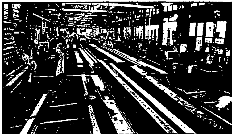
Local 486 Members fabricated all the structural steel for our new International Headquarters Building at the Ingalls Steel Corporation in Washington, D. C.
