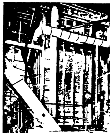
Fig. 3—Walls, Ducts, Casings, Drums of Large Boilers Insulated With INSULAG .
