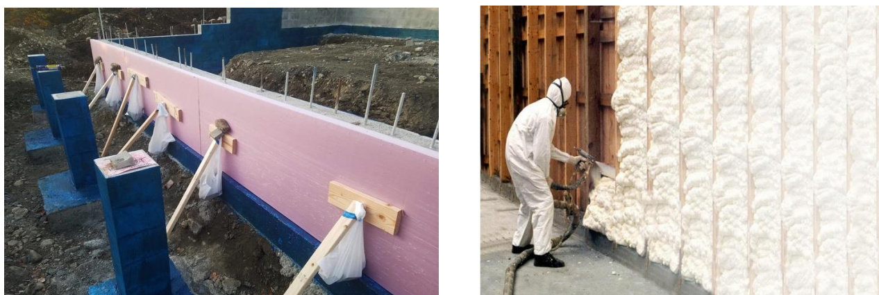
Figure 3. Prefabricated XPS foundation insulation being installed at a building site (left) and direct application of insulating foams (right). Both images used royalty-free from CC BY 2.0, from akhouseproject; and dunktanktechnician.
