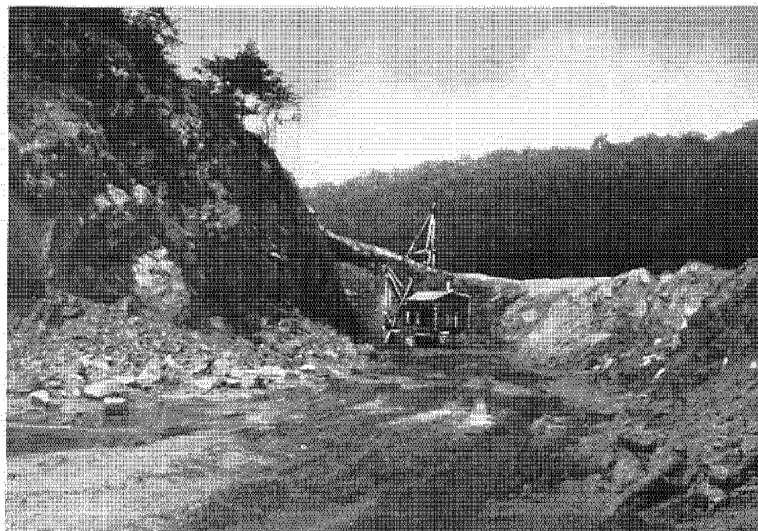
A steam shovel at work on one of the curves cut away in building the road to the river
