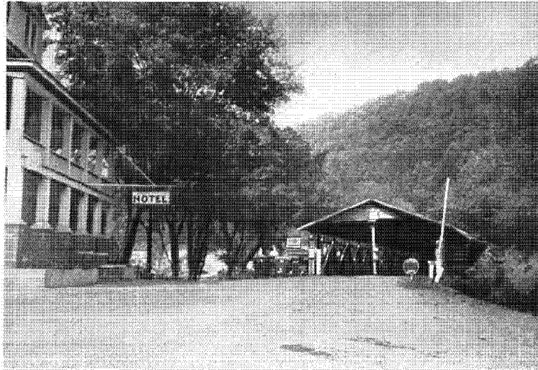
Entrance to the old wooden bridge, looking east
