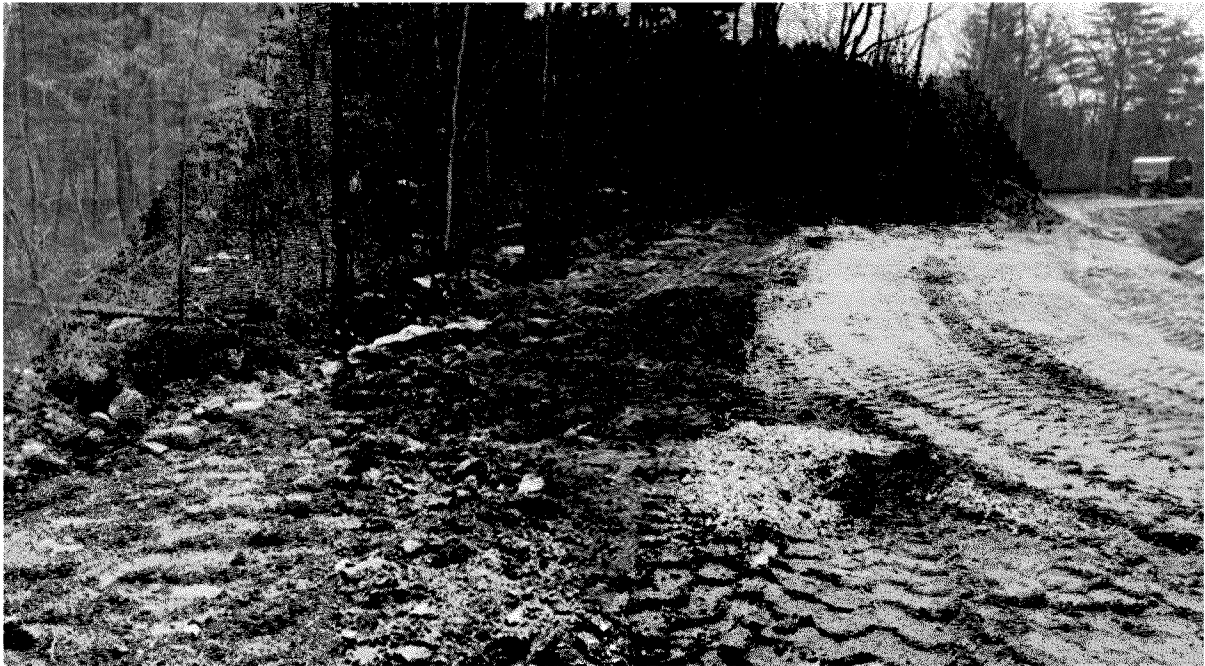
Description: Berm structure continues
