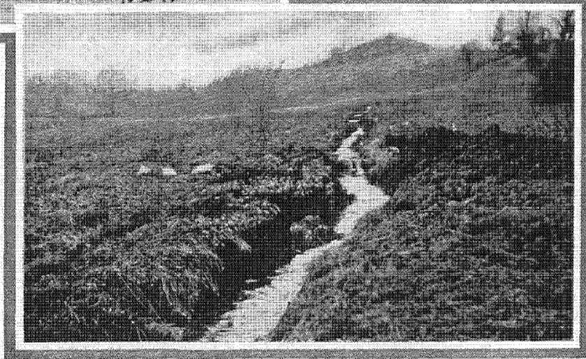
Field After Draining by Use of Dynamite
