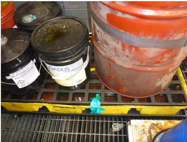
Photo 5: Secondary containment pallet beneath oil product containers near the door of the Scrap Room. The pallet was nearly full of liquid.
