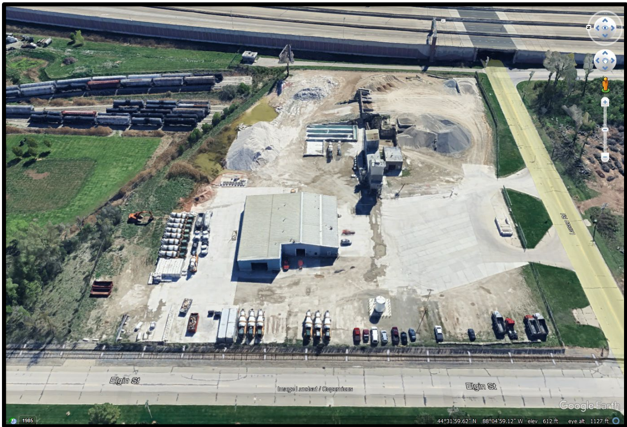
Exhibit 1 : LYCON, Inc. Plant #31, facing east; Source : Google Earth
