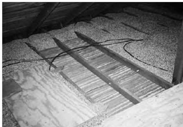
Figure 7—View of ZAI after moving by W.R. Grace & Co. method.
