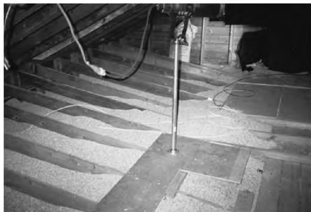
Figure 5—View of attic in home C.
