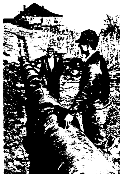
At left, calking part of the 20-in. cast-iron main for Chattanooga, and, at right, water department inspector examining lead-calked lengths of pipe
