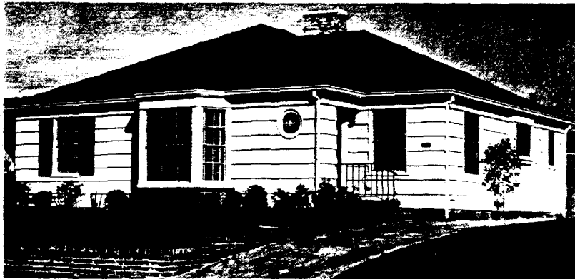
A general view of the new model home, the Certigrade Californian, built of a variety of woods, featuring red cedar shingles painted with white lead
