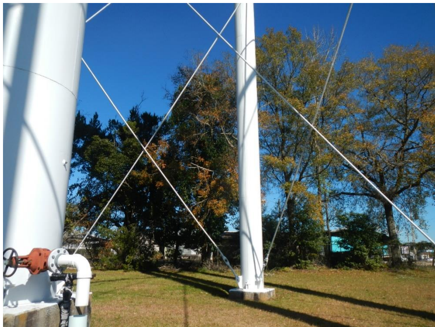
Photograph 8: Vegetation in the vertical plane at Roberts elevated storage tank.
