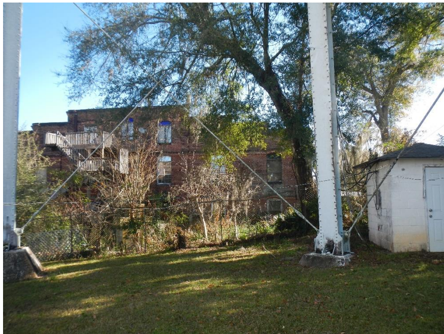
Photograph 20: Live electrical wire extending across the site of Adams elevated storage tank.
