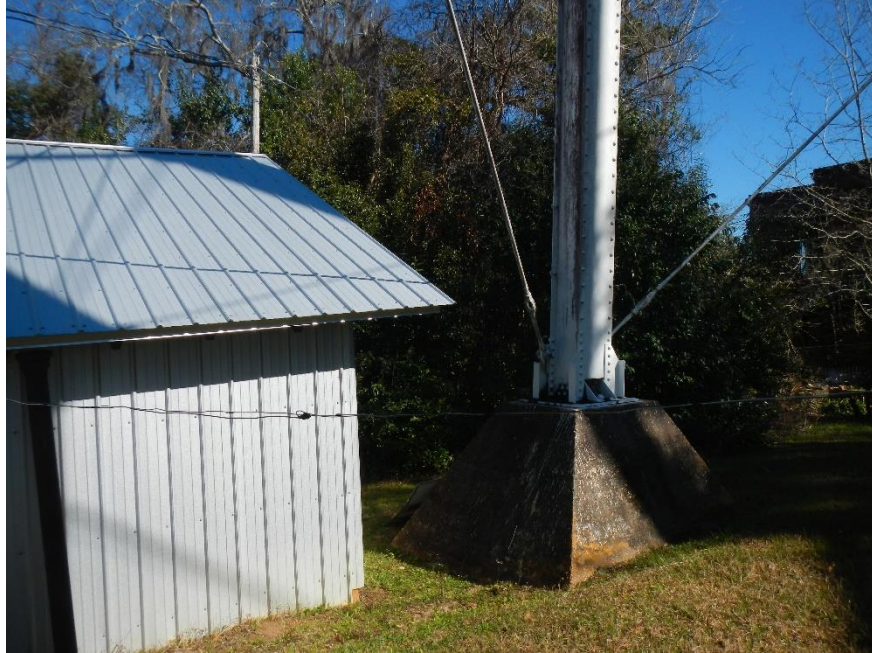
Photograph 21: Live electrical wire extending across the site of Adams elevated storage tank.
