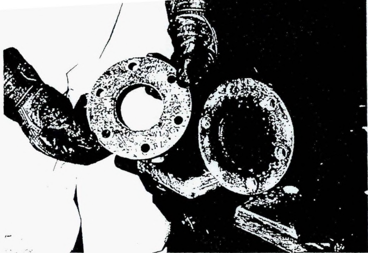
FIGURE 3. After opening the flange, the gasket was first verified as an elastomeric style.
