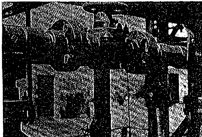
Phenolic CHEMTITE pipe—Hydrochloric Acid—Benzene & traces of Phenol.
