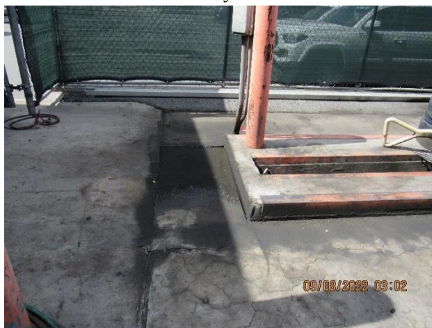
IMG 511 -Evidence of spilled used oil on platform washed-off by stormwater runoff flow away from the used oil storage system.
