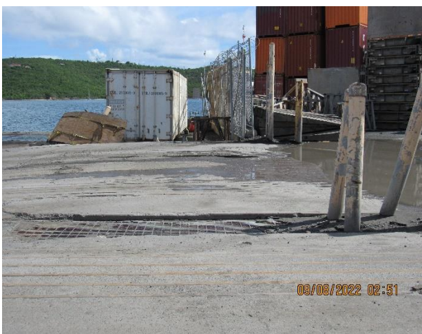
IMG 500 -Large catch basin in which mid-section of the Facility through which stormwater enters the large drainage canal, and into the Bay.
