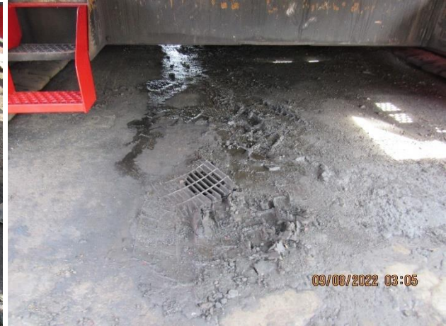
IMG 514 -View of the inlet submerged in oily-mud. Oily-water runoff and sediment entering the Oil/Separator unit. Did not identify discharge port.
