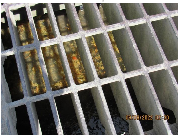
IMG 484 -Close-up view of stormwater catch basin with raised inlet. Observed sea water intrusion with large amount of marine vegetation inside catch basin.
