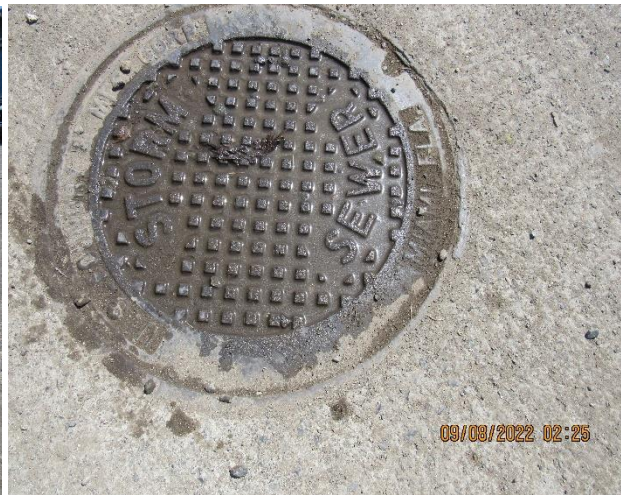
IMG 478 -Picture of cover to storm sewer that conveys stormwater from upstream area.
