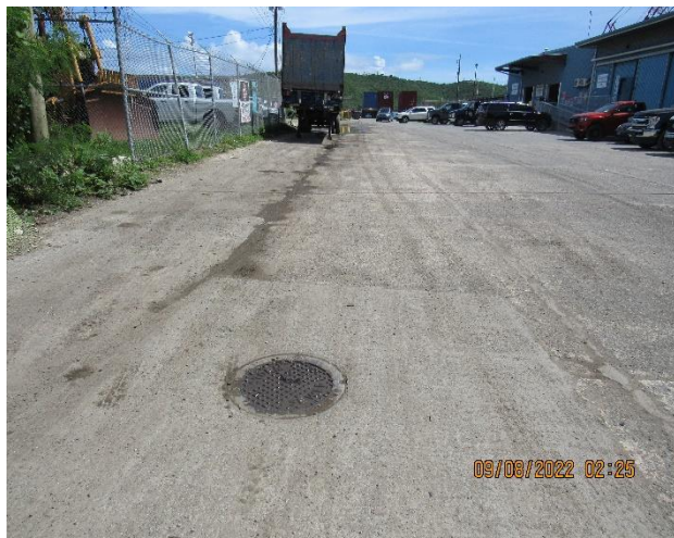
IMG 477 -Road going into the dock area. Sediment transported by storm water runoff from Field seen in the stormwater flow path along the road.
