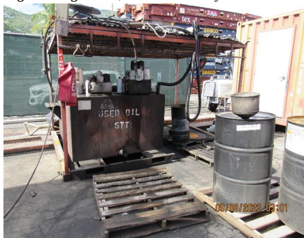
IMG 510 -Use Oil management tank not within containment to capture used oil spills and prevent releases that are exposed to stormwater runoff flow.
