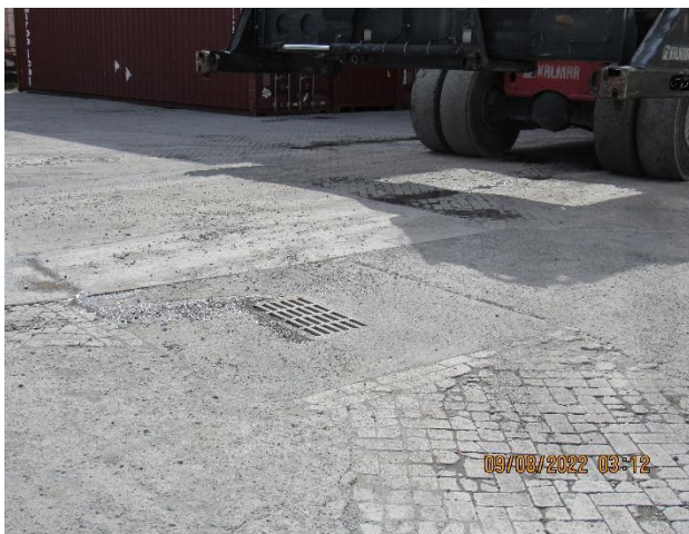
IMG 518 -Stormwater catch basin that drains entire area of Tropical's MT Yard. Inlet of catch basin not protected.
