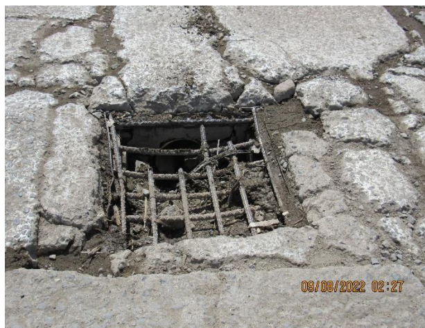
IMG 480 -Close-up of the stormwater catch basin partially clogged with sediment from upstream. The inlet of the catch basin is not protected.
