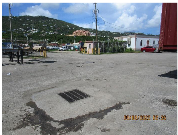
IMG 485 -Stormwater catch basin with raised inlet just in front of Tropical's fenced dock area. The inlet of the catch basin is not protected.
