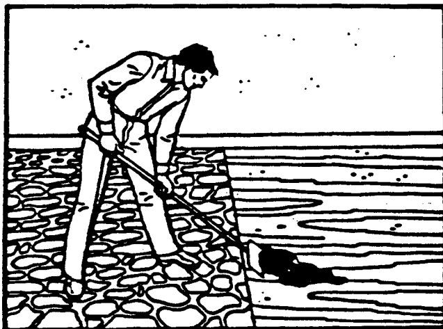
Sketch 13. Stand on the remaining floor covering, not the felt, during felt removal.
