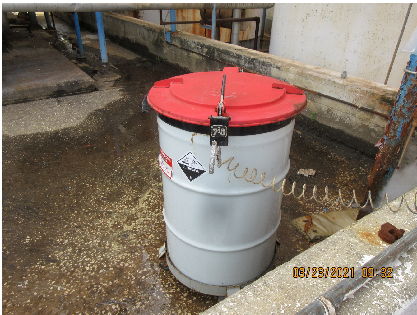
Photo 5 – Drum used to collect filter socks with solidified vapors from the off-loading of materials into tank within the tank farm.
