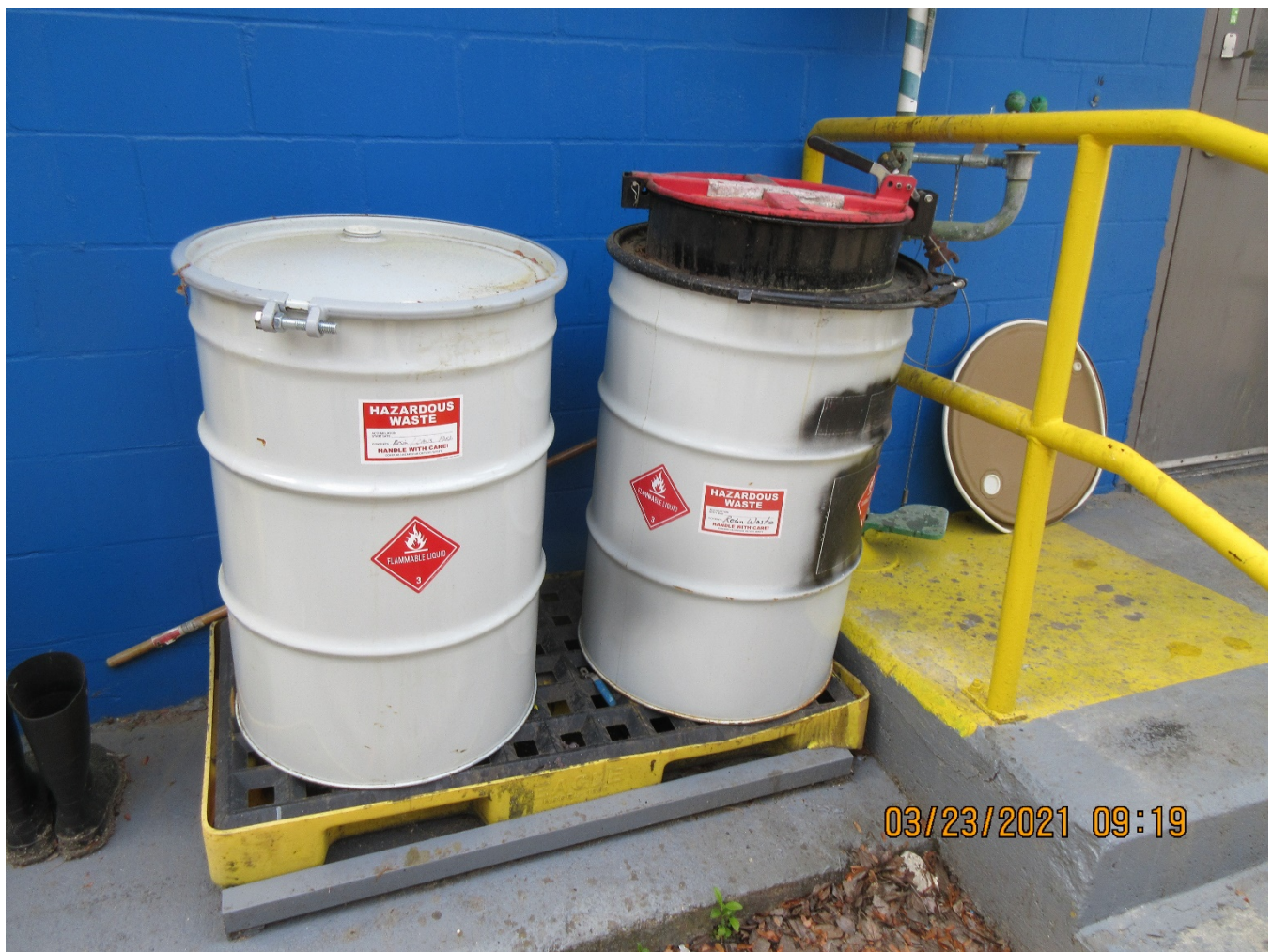
Photo 3 – Hazardous waste collection drums outside of the Production Lab receiving resin and resin cans used for holding samples.
