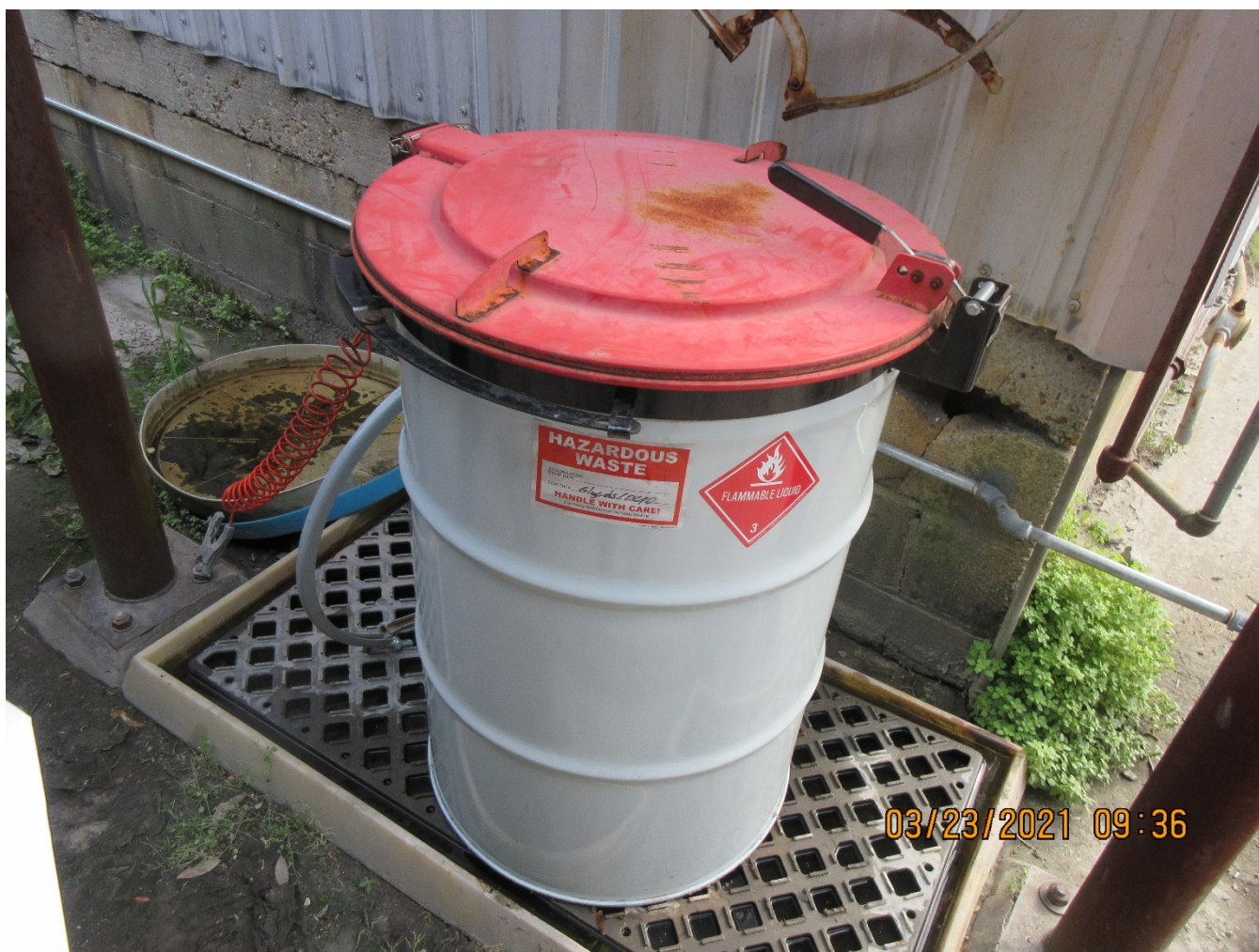
Photo 6 – Drum used to collect DCPD from hose cleanouts in the Rail Car off-loading area.
