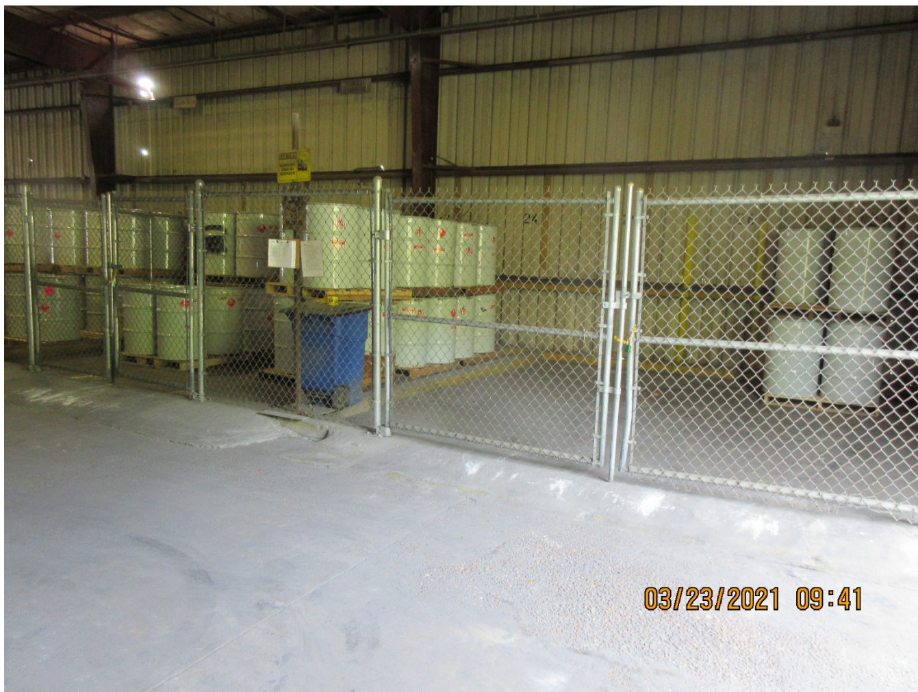
Photo 7 –Hazardous Waste Container Central Accumulation Area
