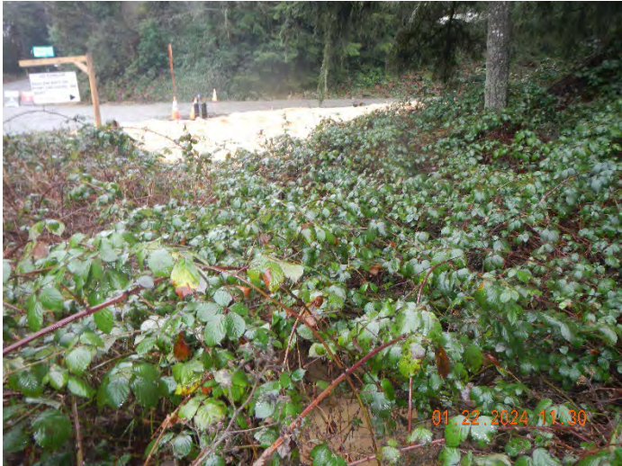
Photo #:04 (DSCN3513) Description: Facing south/southeast, photo of the observed trench dewatering discharge location. A vegetative area on the north side of SW Birt Drive, south of SR-3 along Sunnyslope Road SW.
