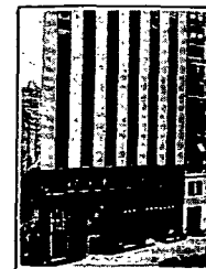
Fourteen Stories of this Building at 28 East 40th Street, New York City, are Air Conditioned with Frick Freon-12 Refrigeration
