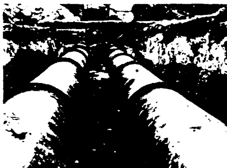
U. S. PIPER Lead calked cast-iron gas lines from producer to purifier in an eastern gas plant.
