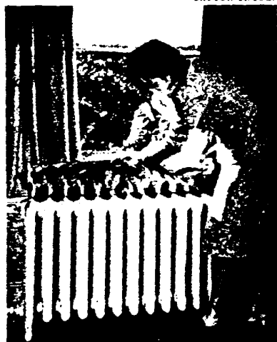
Placing lead foil reflective insulation behind radiator.
