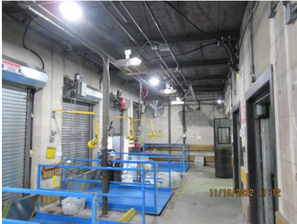
Photograph #3 – Loading Dock
