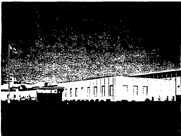
Ground level view of the company's new floor tile plant at Hayward, California.
