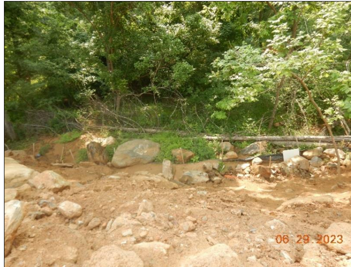
Rosedale Development Site Date: 29 June 2023 Photo ID: DSCN4782.JPG Photo taken by: Katelyn Almeter
