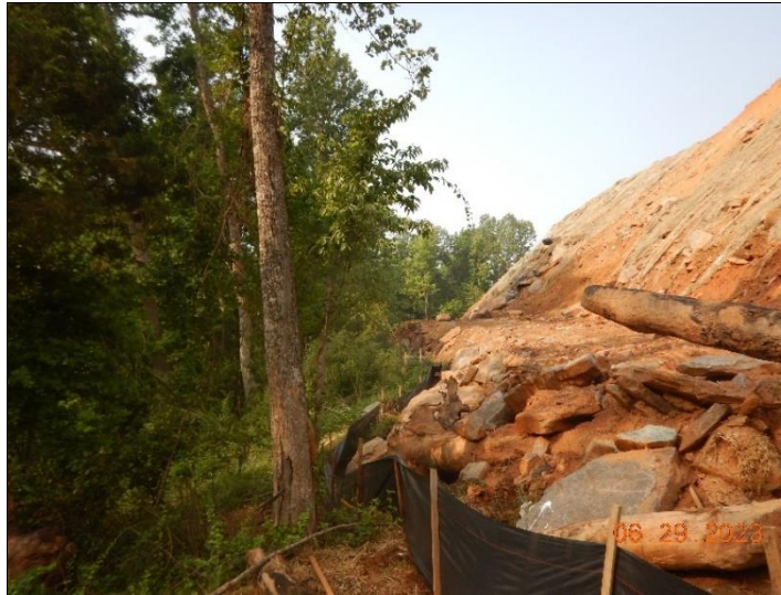
Rosedale Development Site Date: 29 June 2023 Photo ID: DSCN4755.JPG Photo taken by: Katelyn Almeter
