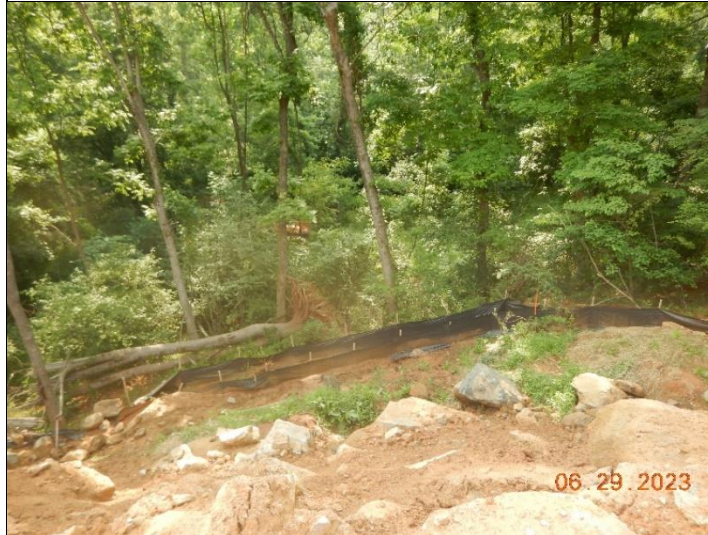
Rosedale Development Site Date: 29 June 2023 Photo ID: DSCN4784.JPG Photo taken by: Katelyn Almeter
