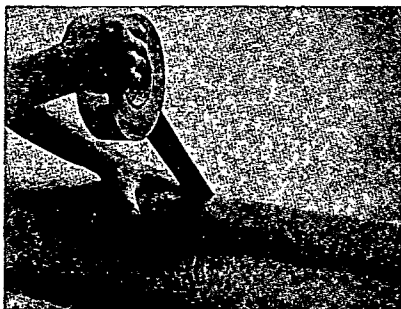
J-M Micro-Aire duct sections have factory-formed "slip joints" for strong, snug connections. Tight seal is completed with pressure-sensitive tape.
