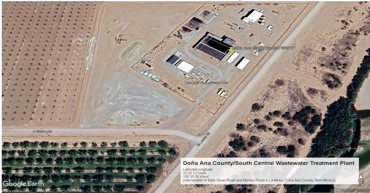
Aerial Image #1- Doña Ana County/South Central Wastewater Treatment Plant
