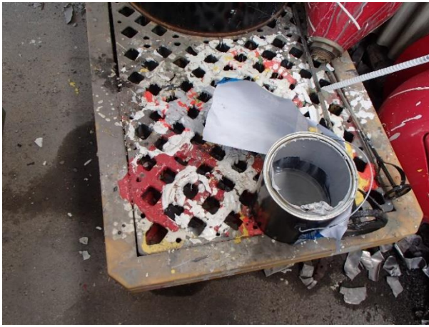
Photo 12: Building 134 Waste Paint SAA container spill pallet.
