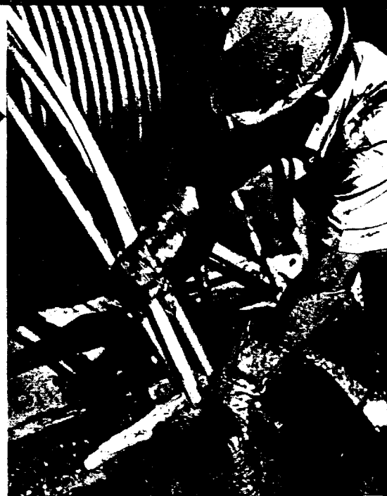
Workman strapping neutral conductor onto pulling eye for easy pulling into conduit.
