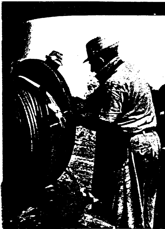
Crossed bars at tube mouth prevent the cable from twisting within the conduit.
