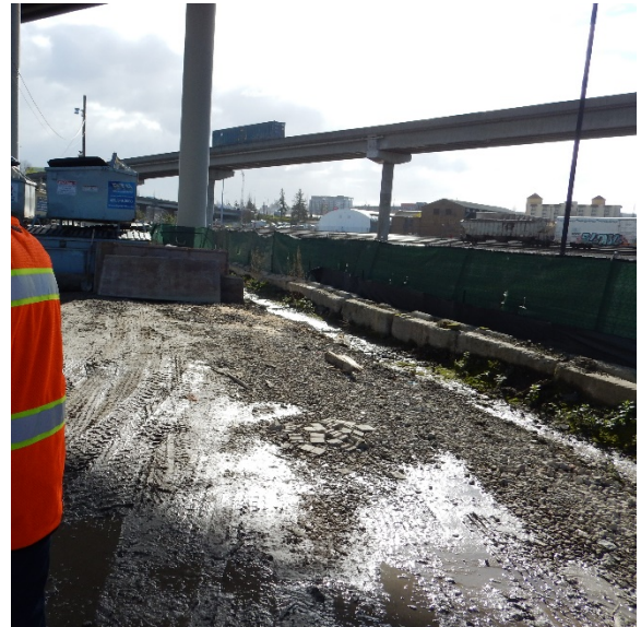
Photo #:06 (DSCN0755) Description: Facing south, photo of stormwater collecting in a shallow trench. Note the concrete blocks bordering the trench and property line.
