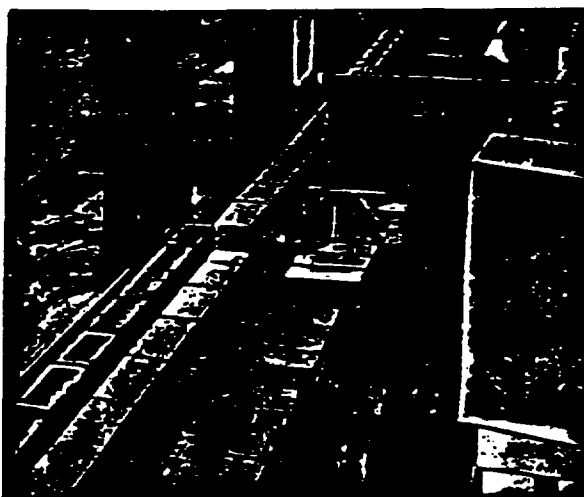
Outside wall of Cross Cracking Unit being insulated with 4\frac{1}{2} " of Sil-O-Cel C-22 Brick in "core wall" construction
