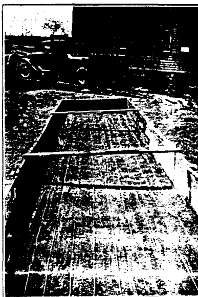
Heating cables laid out on the sand, properly spaced
