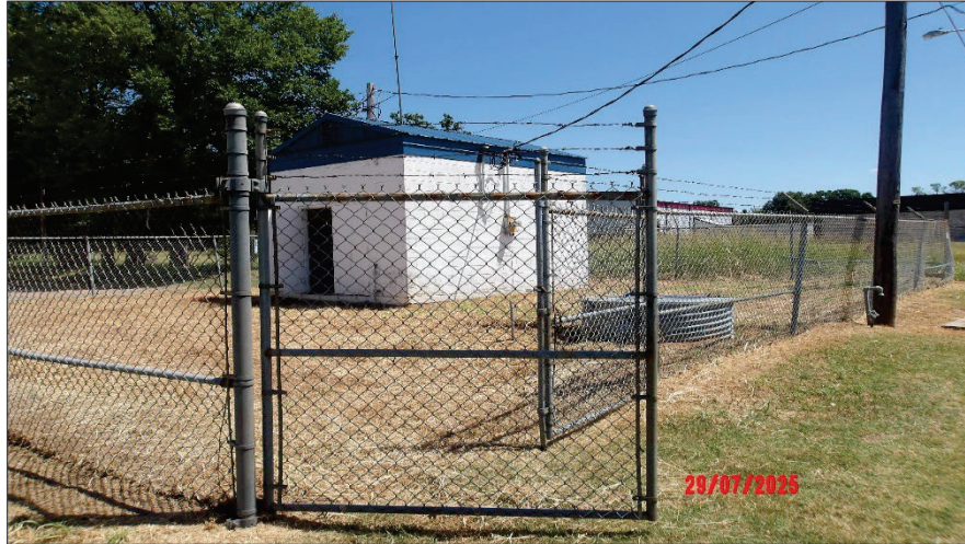
Photograph 77. 7/29/2025 13:55 100_0231.JPG North Highway 81 Pumphouse Description: Security fencing at North Highway 81 Pumphouse missing proper signage.
