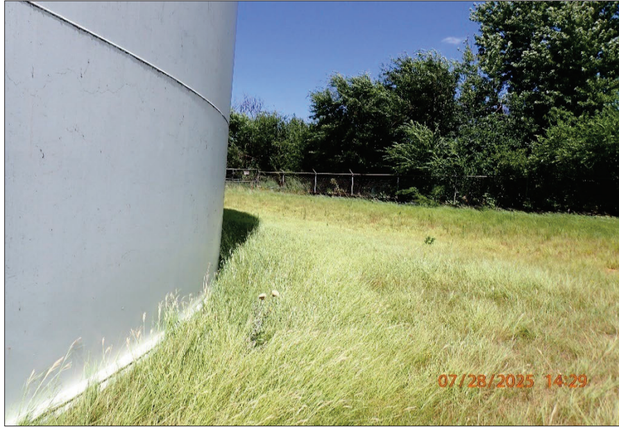
Photograph 57. 7/28/2025 14:29 P7280096.JPG El Rancho Tower
