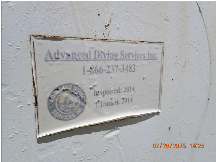
Photograph 56. 7/28/2025 14:25 P7280086.JPG El Rancho Tower
