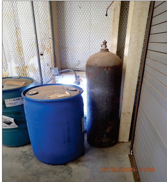
Photograph 29. 7/29/2025 10:39 P7290448.JPG Ammonia Storage Room
