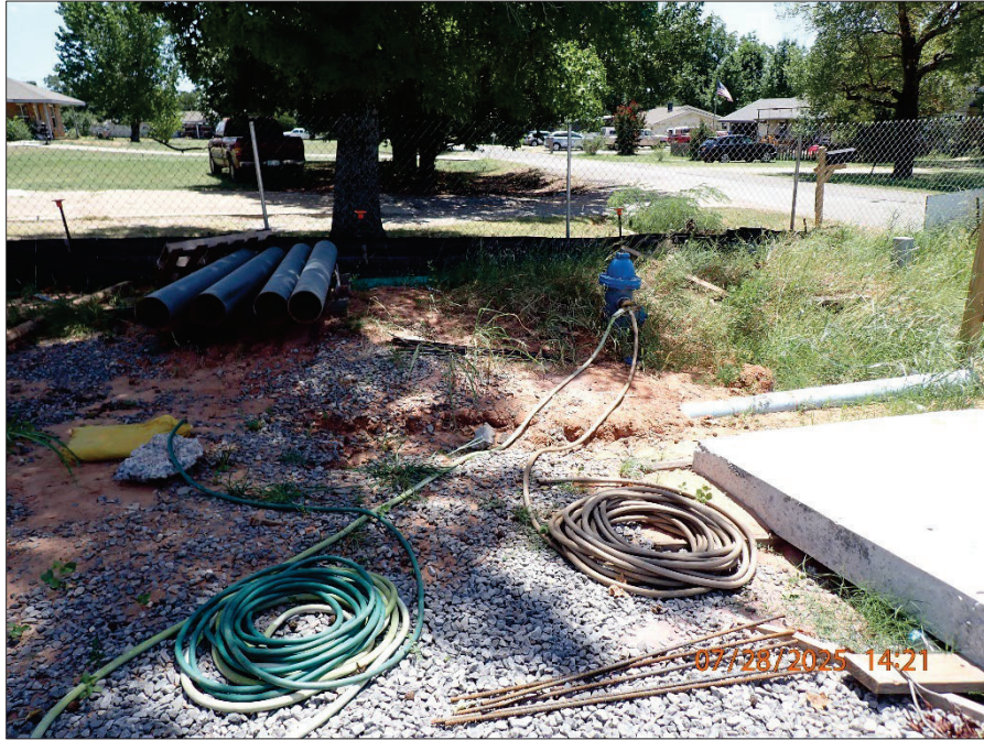
Photograph 55. 7/28/2025 14:21 P7280076.JPG El Rancho Tower
