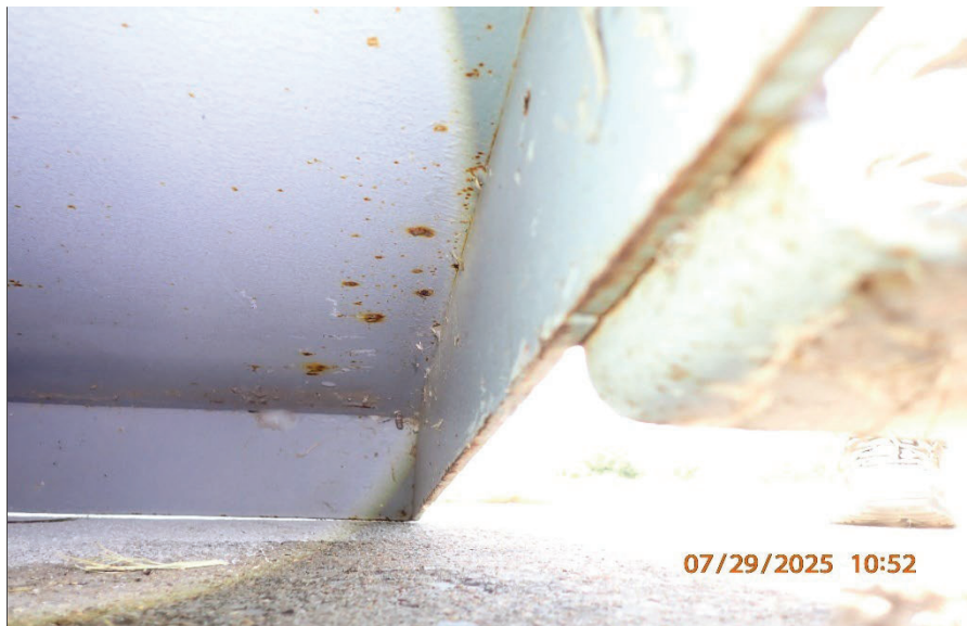
Photograph 32. 7/29/2025 10:52 P7290484.JPG 3.5 MG Clearwell
