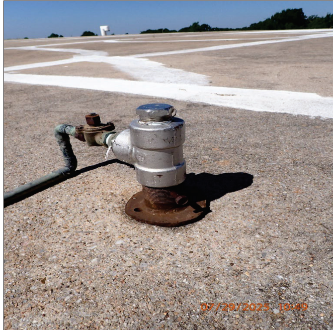
Photograph 35. 7/29/2025 10:49 P7290477.JPG 3.5 MG Clearwell
