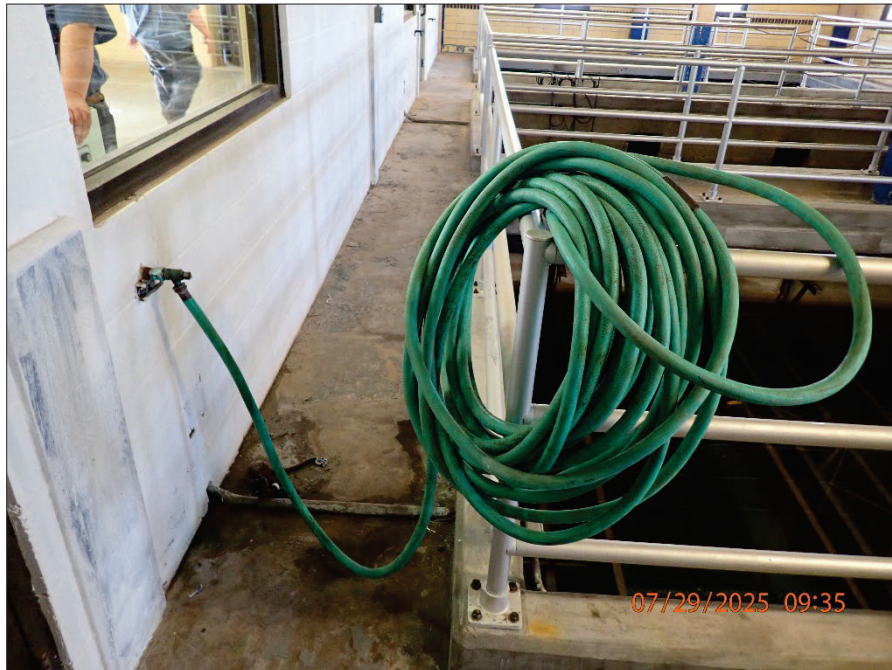
Photograph 9. 7/29/2025 09:35 P7290322.JPG South Plant Filter 1 & 2
