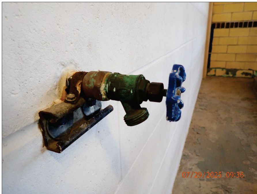
Photograph 10. 7/29/2025 09:36 P7290328.JPG WTP South Plant Filter
