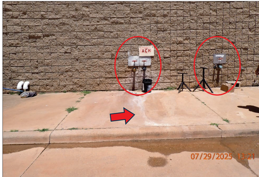
Photograph 45. 7/29/2025 13:21 P7290544.JPG WTP Chemical Loading Zone
