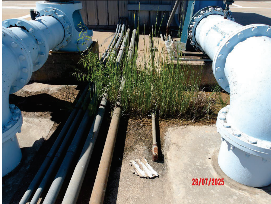
Photograph 37. 7/29/2025 09:58 100_0115.JPG 3.5 MG Clearwell
