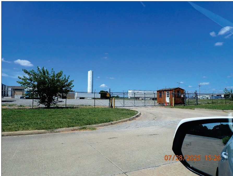
Photograph 72. 7/28/2025 15:26 P7280192.JPG North Industrial Tower #1 (West) Description: Security fencing blocking access to North Industrial Tower #1 (West).
