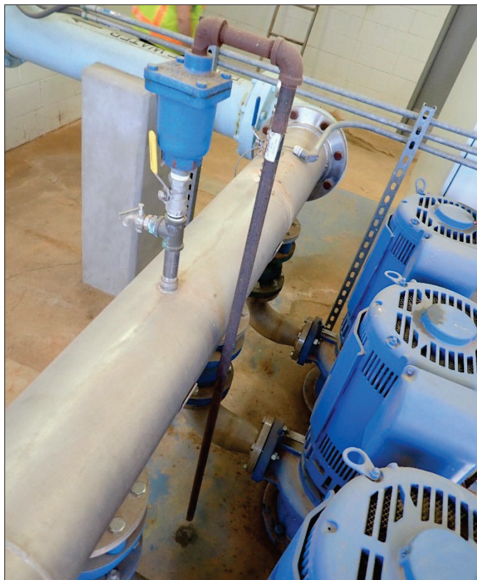
Photograph 60. 7/28/2025 15:11 P7280187.JPG 10th and Elk Pumphouse
