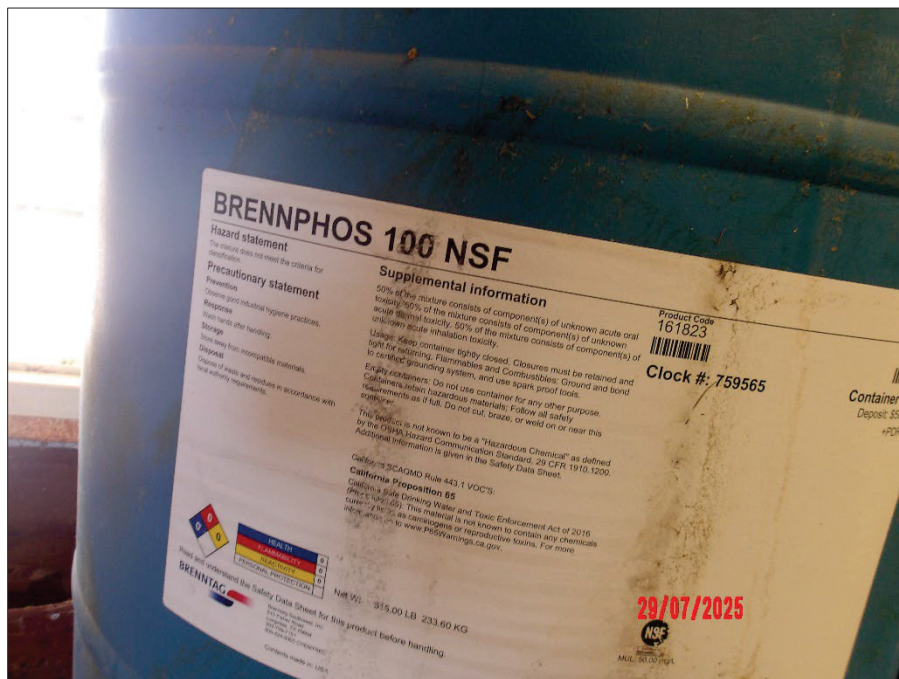
Photograph 25. 7/29/2025 09:41 100_0103.JPG Ammonia Storage Room
