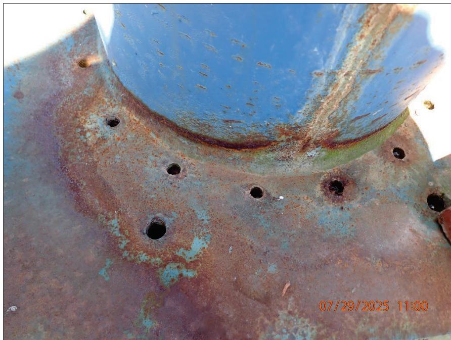
Photograph 38. 7/29/2025 11:00 P7290503.JPG 3.5 MG Clearwell
