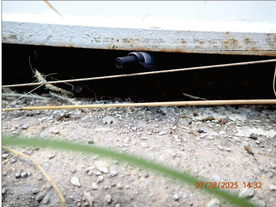
Photograph 59. 7/28/2025 14:32 P7280106.JPG El Rancho Tower
