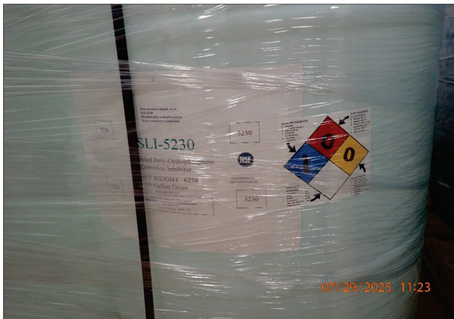
Photograph 39. 7/29/2025 11:23 P7290518.JPG Polyphosphate Storage Room Description: Drums of blended poly-orthophosphate corrosion control inhibitor stored in the WTP Polyphosphate Storage Room.
