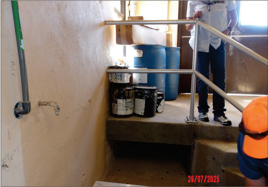
Photograph 12. 7/29/2025 08:57 100_0044.JPG South Plant Filter Gallery
