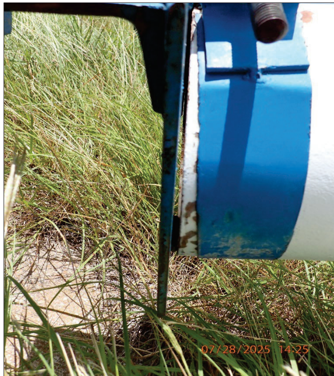
Photograph 58. 7/28/2025 14:25 P7280090.JPG El Rancho Tower
