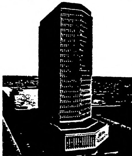
In Los Angeles—The California Federal Plaza building roof serves as a landing spot for helicopters. For waterproofing under the helistop slab, Charles Luckman Associates, architects, selected a Koppers 5-ply coal-tar pitch waterproofing membrane. A similar system protects the 4th floor roof, under a slate promenade. On the ground, twenty large planting boxes are waterproofed with a similar 3-ply built-up membrane covered with ½" insulation for protection from the dirt. Basement walls outside a service and storage area are kept permanently dry with a Koppers system of priming oil plus a 3-ply waterproofing membrane and a top coating of pitch.
