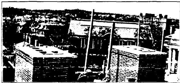
Two lead covered chimneys with rain-water vents
