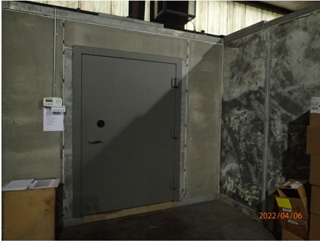
Photo 9: DEA Controlled Substances Vault.
