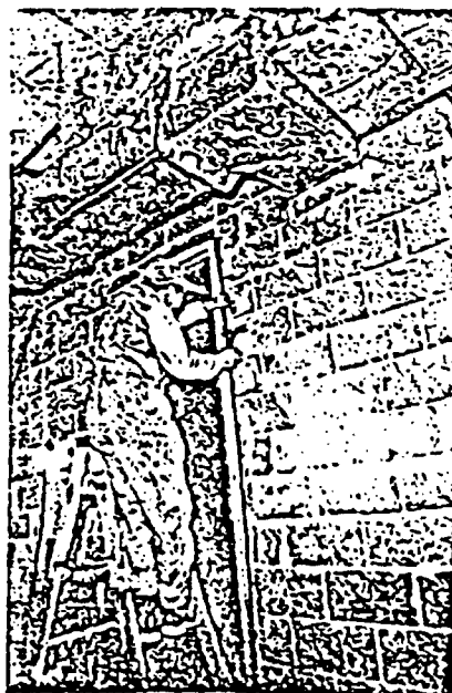
• LATHER PUTS on CAB around door opening for "shadow detail."
