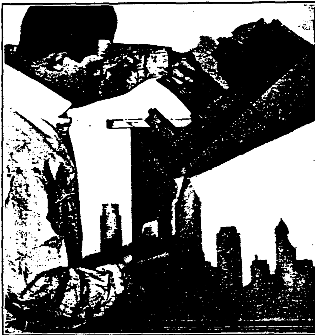
Part of frisket raised to show section of wall on which skyline design has been applied
